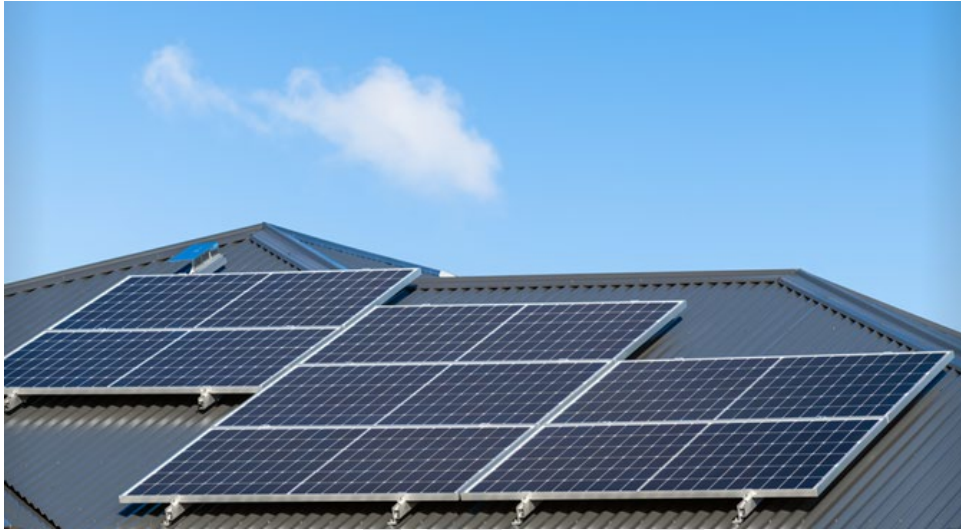
Figure 6 – Typical rooftop solar panel system
