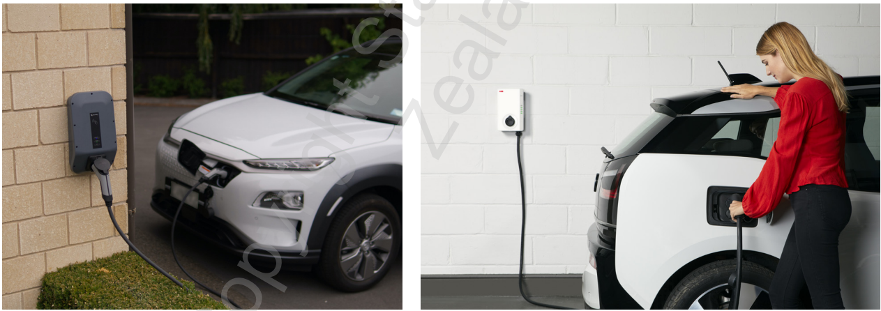
Figure 12 – Positioning EVSE in a car port or off-street parking location
