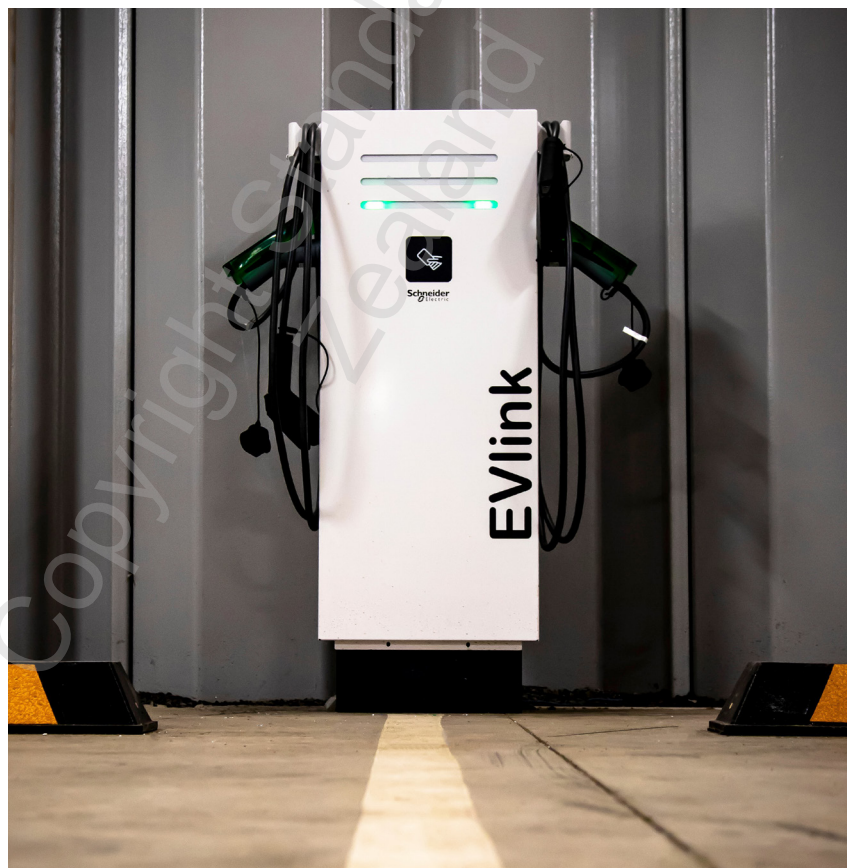
Figure 13 – Mode 4 (DC) 24 kW pedestal charging stations
