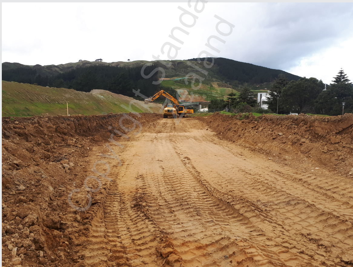
Figure 7 – Example of weaving in clay fill
