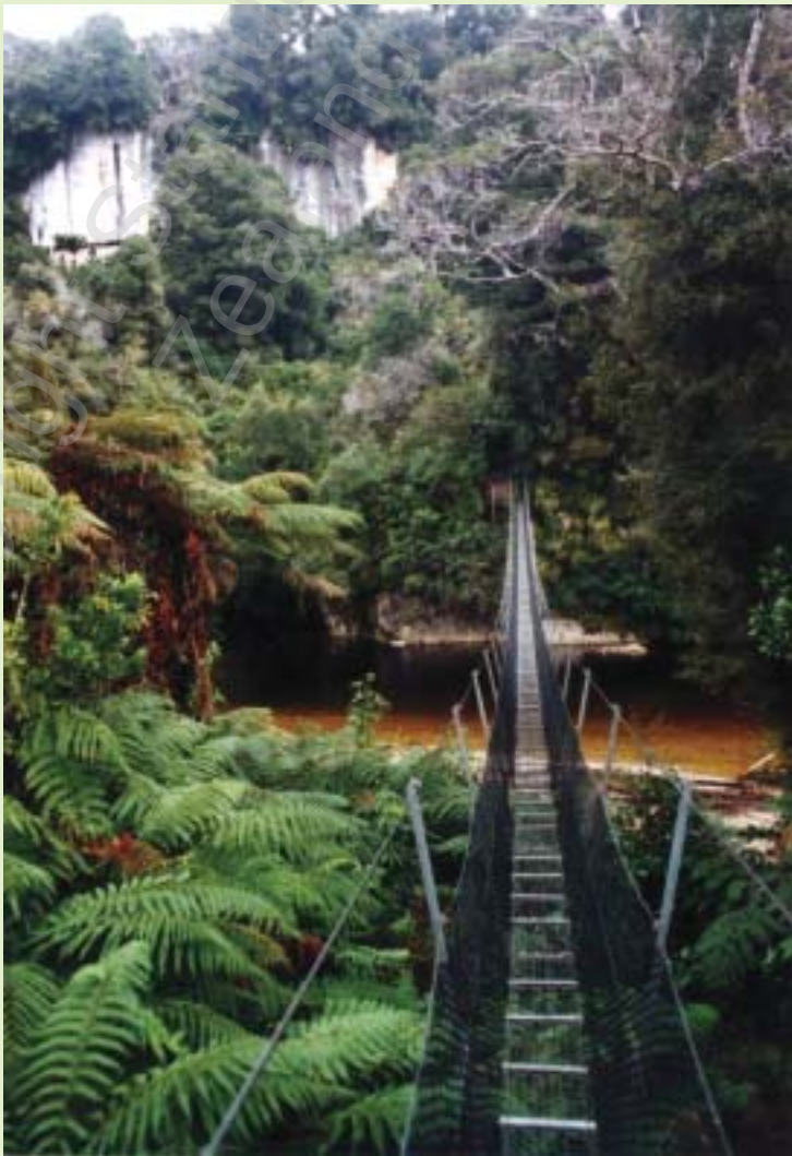
Figure 12 – Bridge over Heaphy River
