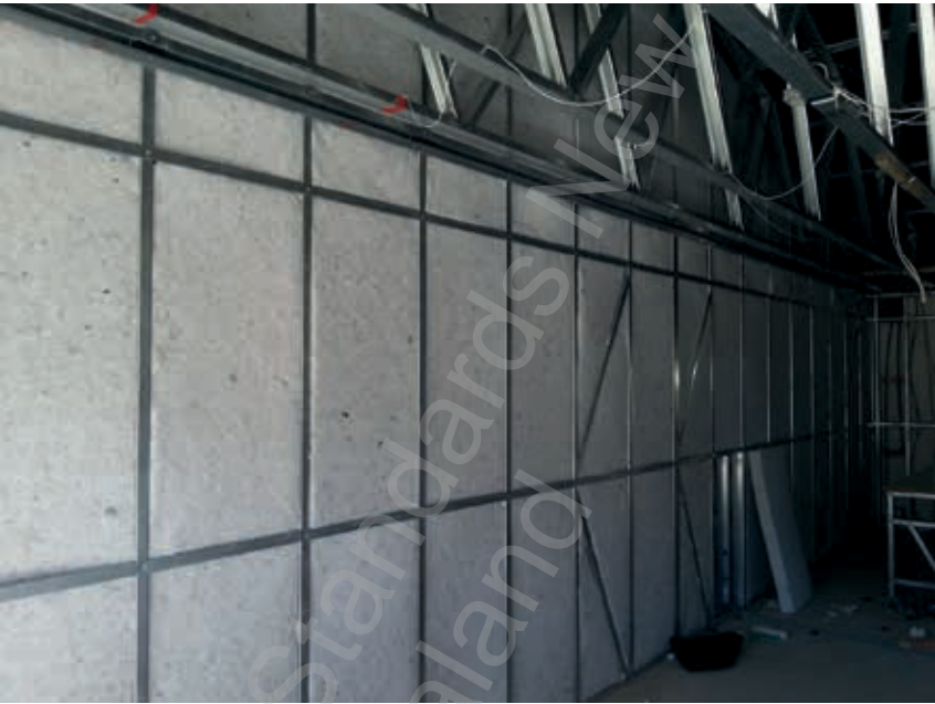
Figure 16 – Insulation fitted into a steel-framed wall
