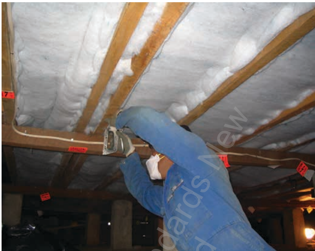
Figure 30 – Installed underfloor blanket
