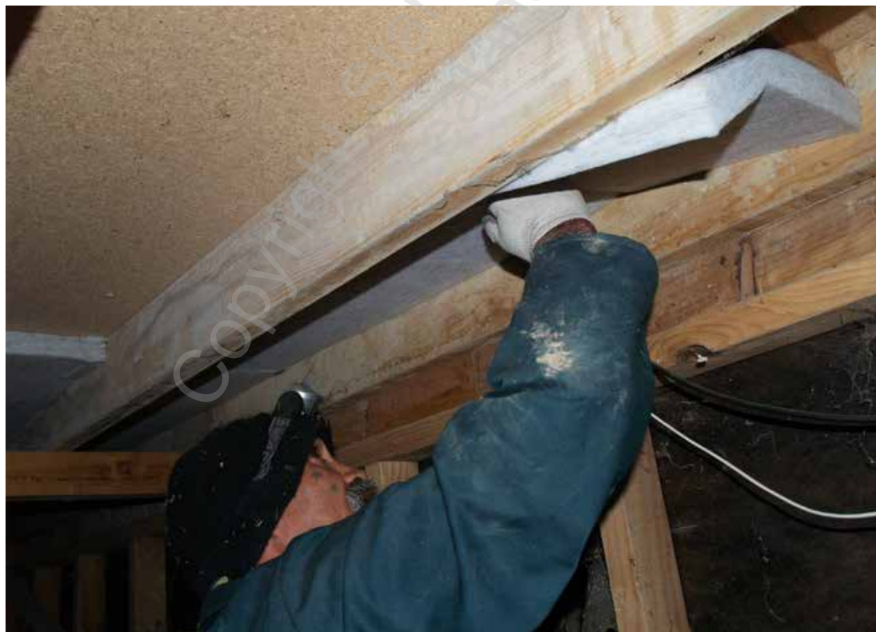
Figure 32 – Fitting semi-rigid sheets
