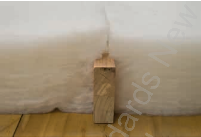
Figure 29 – Friction-fitting insulation over joists
