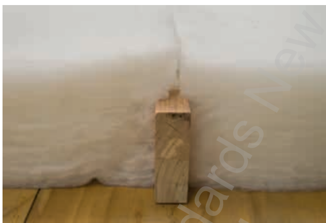
Figure 29 – Friction-fitting insulation over joists
