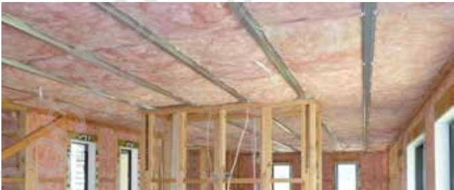
Figure 27 – Segments installed in a ceiling
