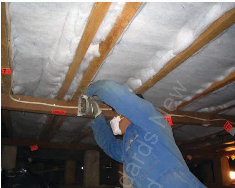
Figure 30 – Installed underfloor blanket
