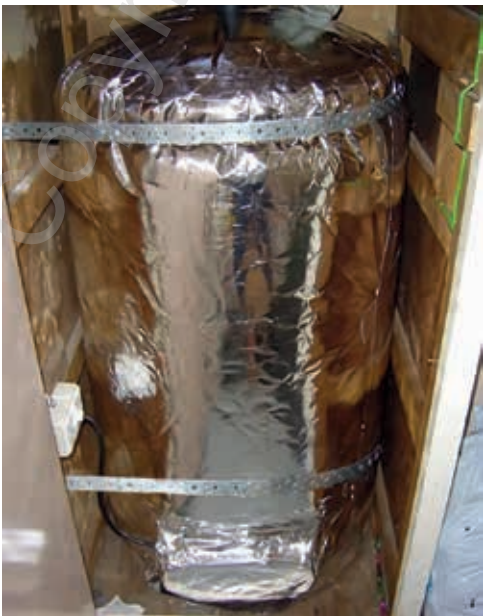
Figure 35 – Insulated hot water cylinder
