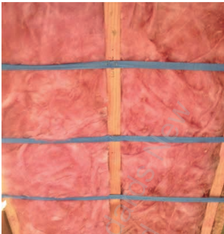
Figure 28 – Blanket in a ceiling secured with strapping
