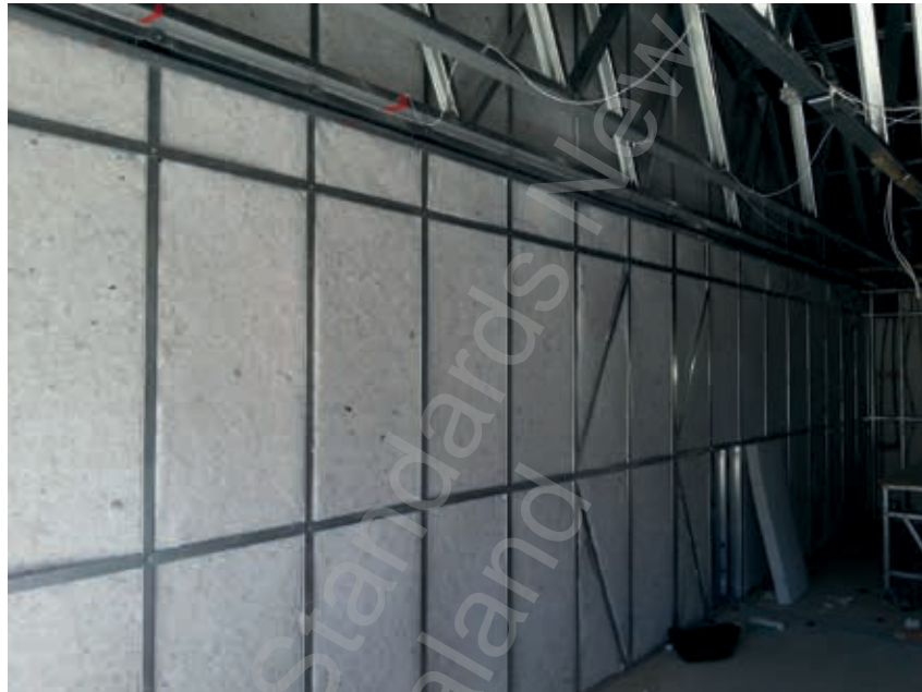
Figure 16 – Insulation fitted into a steel-framed wall
