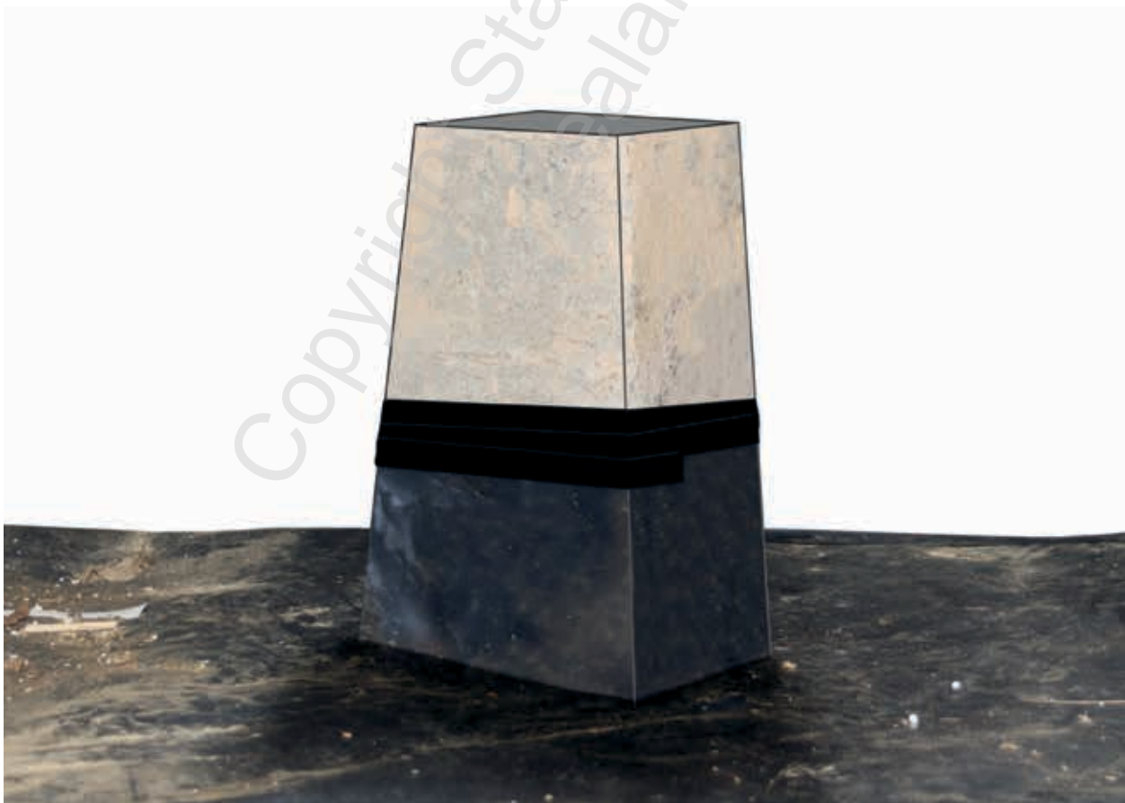
Figure 34 – On-ground vapour barrier folded up and taped around a pile
