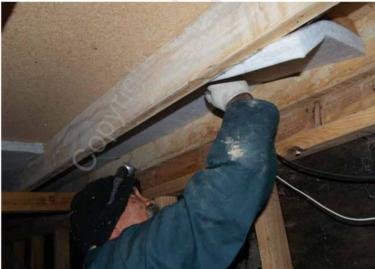
Figure 32 – Fitting semi-rigid sheets
