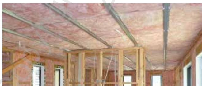
Figure 27 – Segments installed in a ceiling
