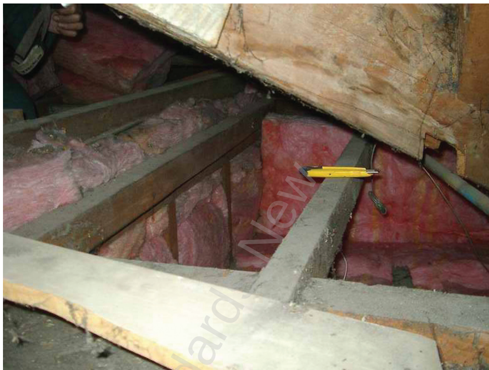
Figure 2 – Recessed ceiling space
