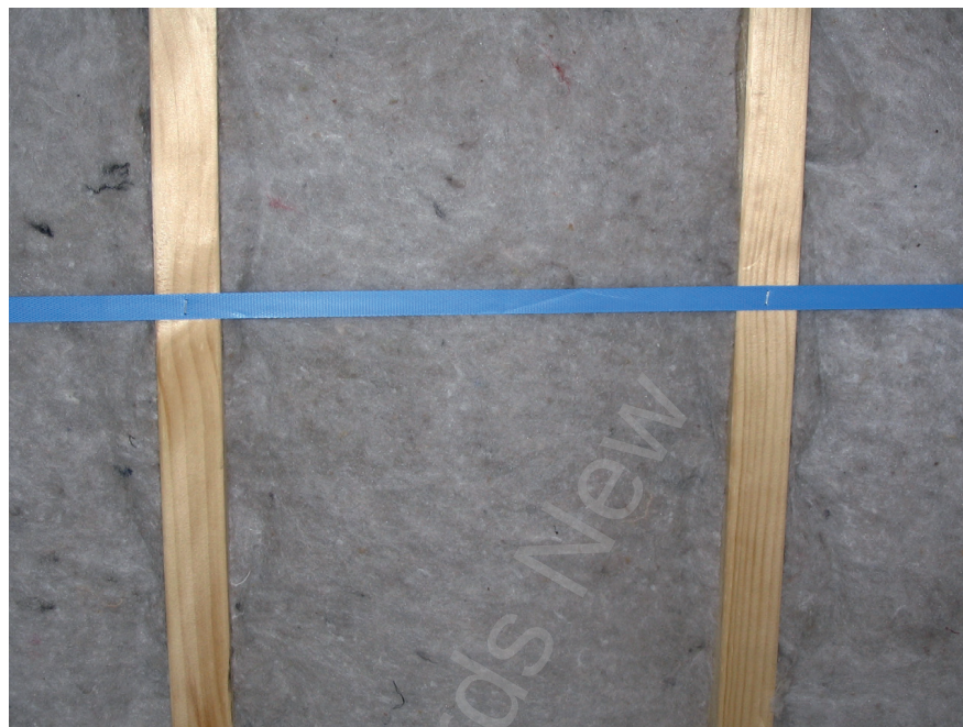
Figure 5 – Blanket in ceiling secured with strapping
