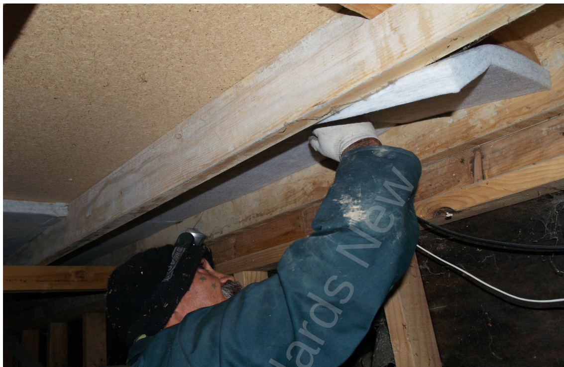
Figure 16 – Fitting semi-rigid sheets
