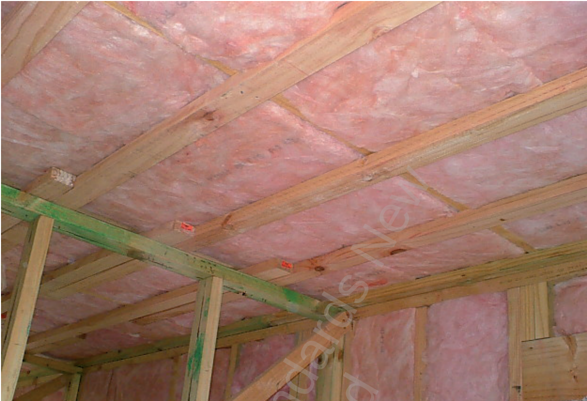
Figure 4 – Segments in unlined ceiling
