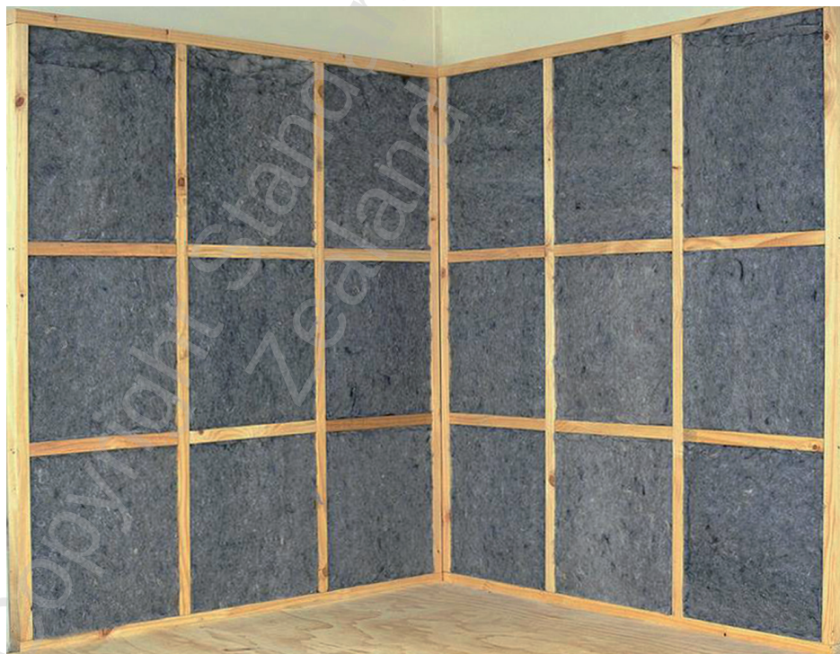
Figure 13 – Completed blanket installation in framed walls
