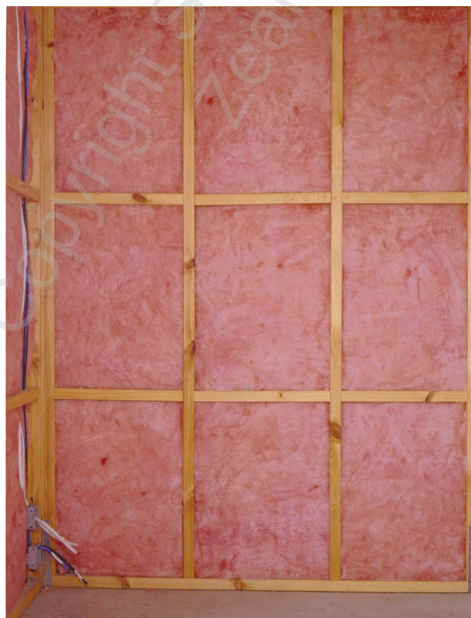
Figure 10 – Segments correctly installed in new wall
