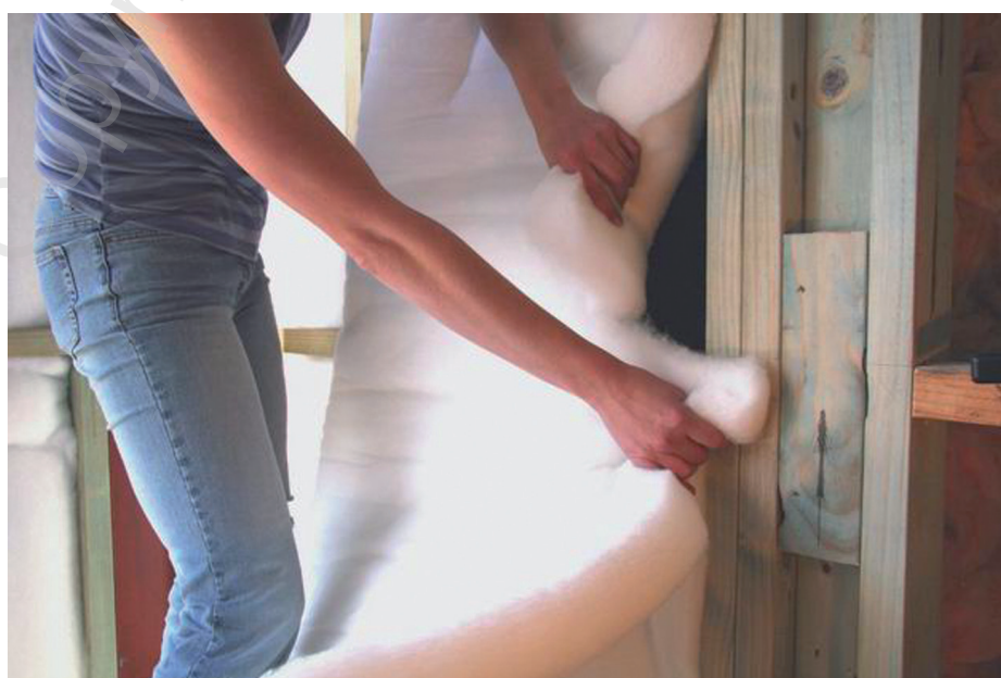
Figure 11 – Tearing blanket to fit
