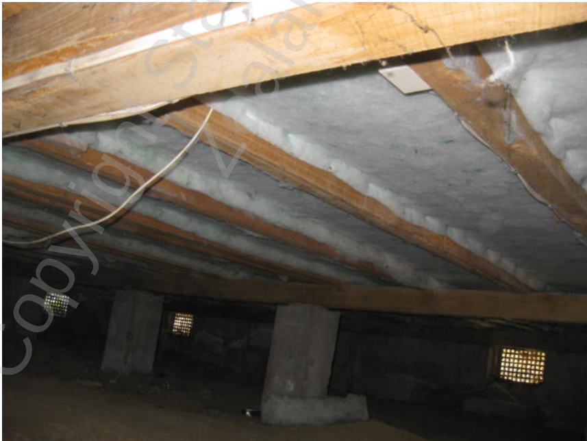
Figure 14 – Installing underfloor blanket
