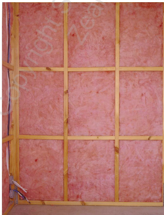
Figure 10 – Segments correctly installed in new wall
