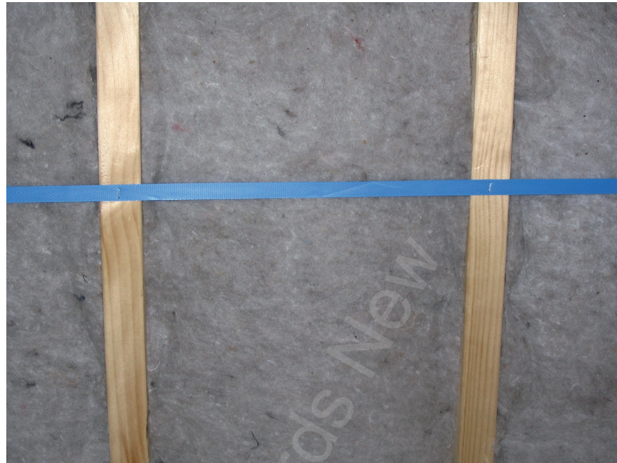
Figure 5 – Blanket in ceiling secured with strapping
