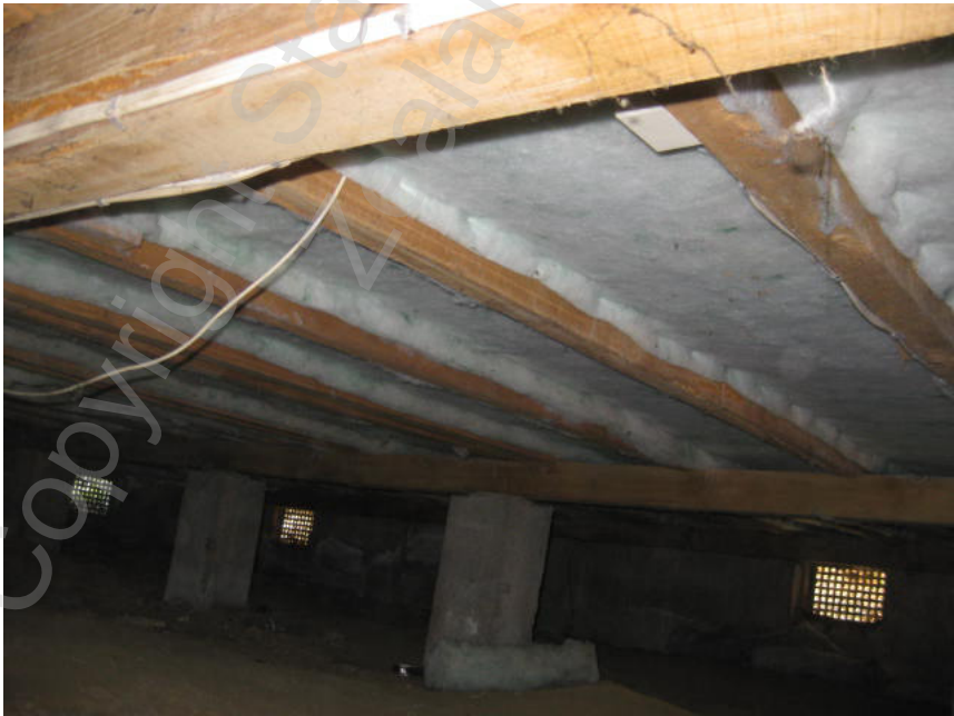
Figure 14 – Installing underfloor blanket
