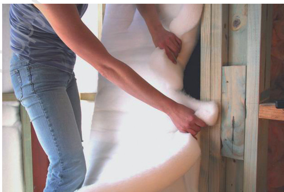
Figure 11 – Tearing blanket to fit
