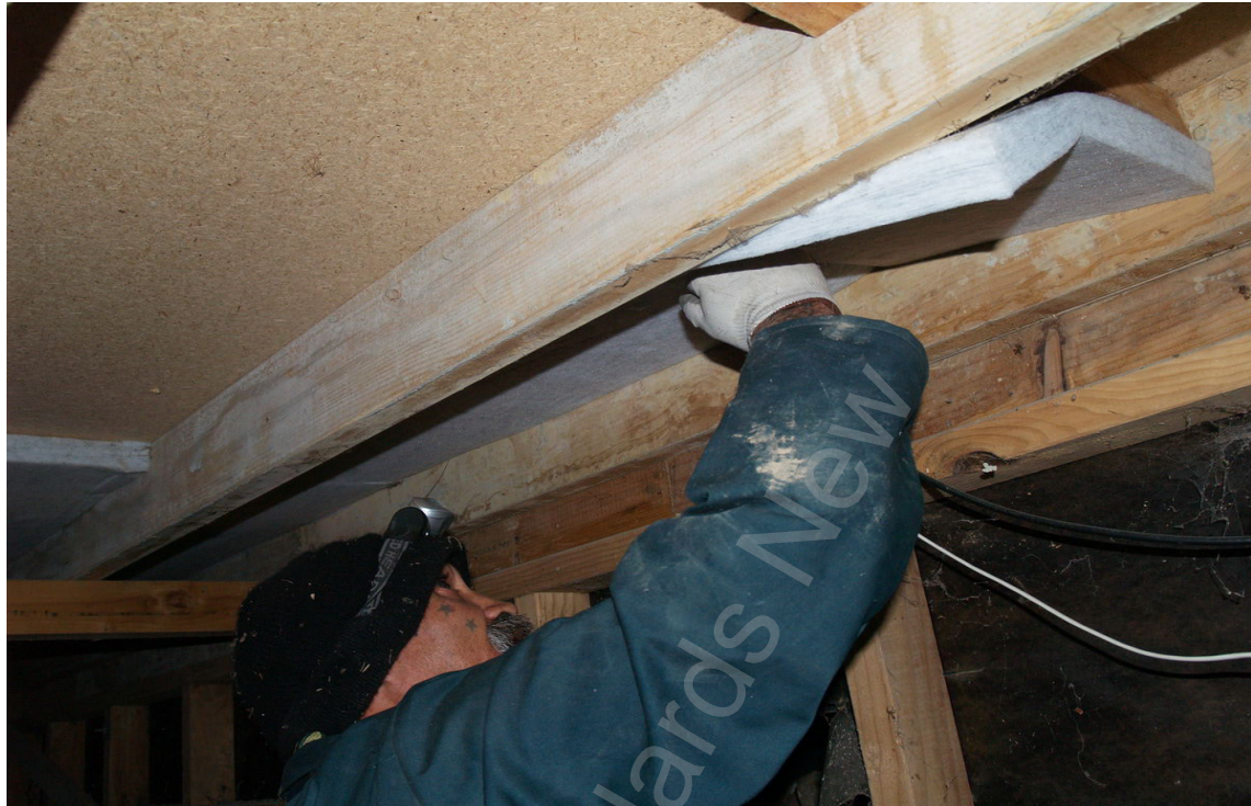
Figure 16 – Fitting semi-rigid sheets
