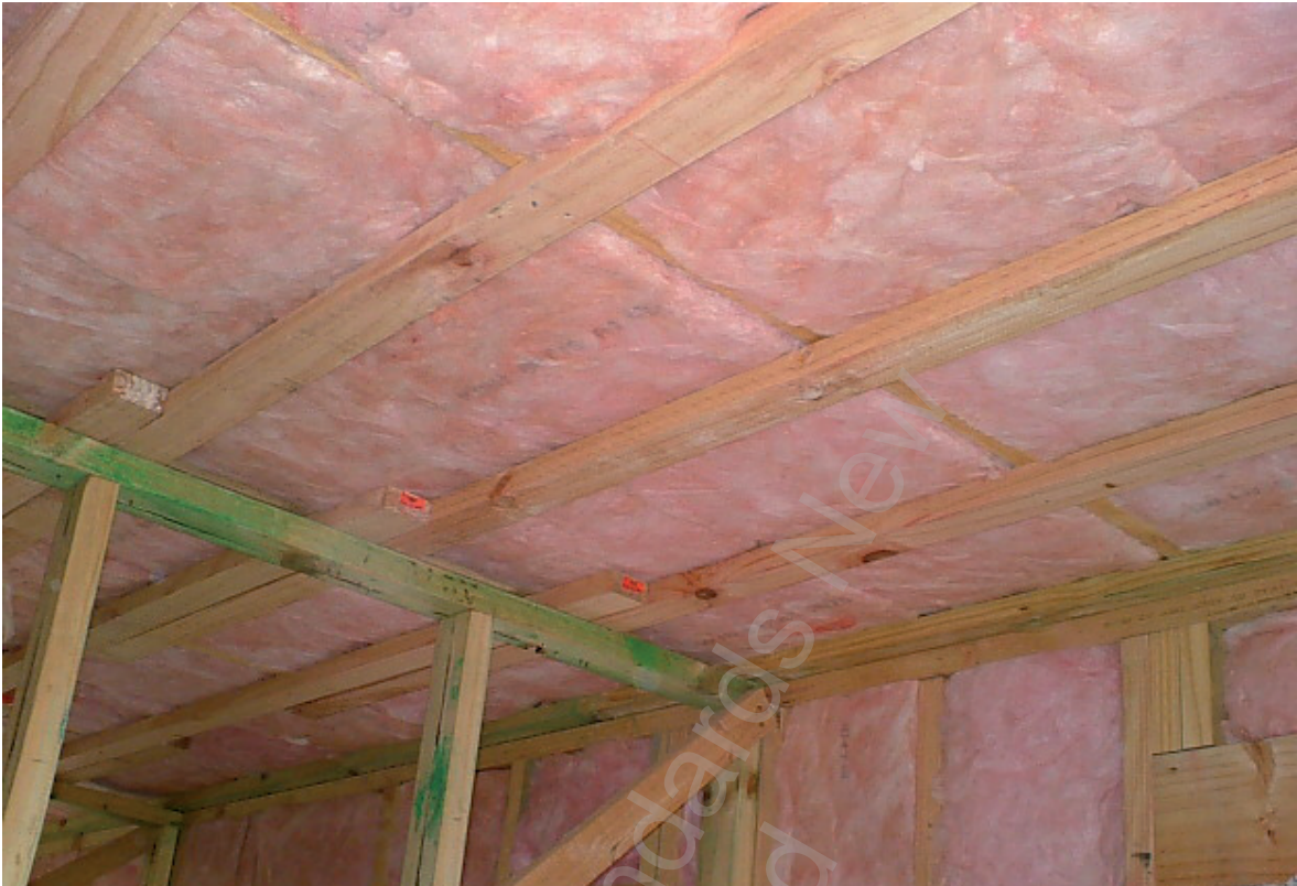
Figure 4 – Segments in unlined ceiling
