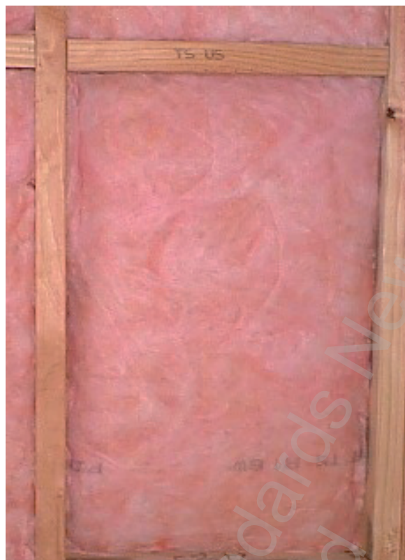
Figure 9 – Example of ‘tucking in’ showing undesirable compression of insulation at edges
